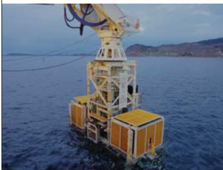
Figure 7. Remote Tee Welding Tool.
