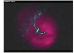
Crack viewed under UV
