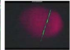
Crack viewed under UV
